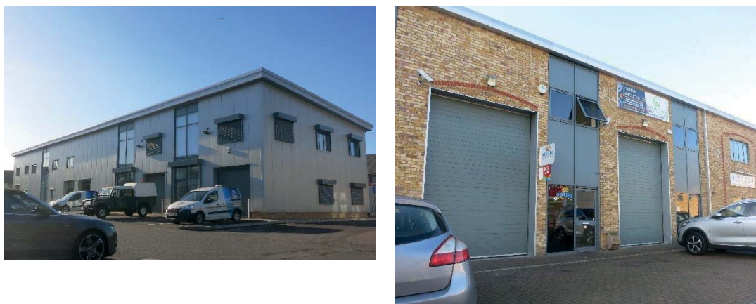
Figure 4.3 The Foundry (left), Eurocentre (right)
