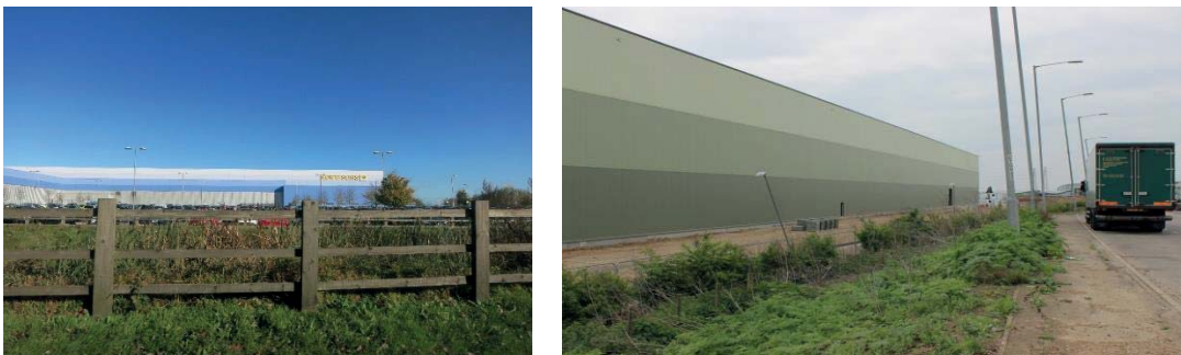
Figure 4.7 Morrisons Distribution units (G-Park) & Aldi Distribution unit
